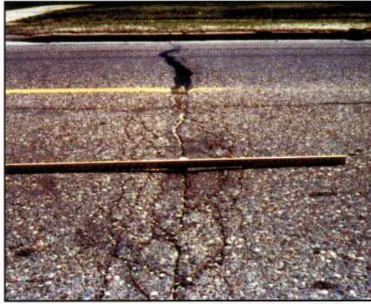
The far side of this asphaltic concrete pavement was sealed by SAMI Road Services. The treated crack shows no signs of further deterioration. As you can see on the untreated near side of this pavement, there is extensive cracking and deformation.
