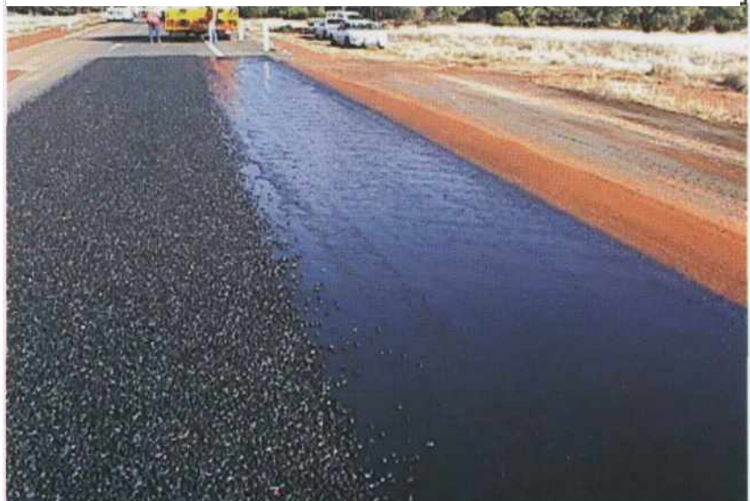
These photos show the transformation of one section of Queensland DMR's Warrego Highway project. The top photo shows the original cracked seal showing the weak shoulders and wheel path deformation due to heavy rain and traffic. The bottom photo shows the SAMiflex E50 high residue polymer modified emulsion being applied to the full width of the pavement. The shoulders were in-situ stabilised and formation width increased to 9.0m.
