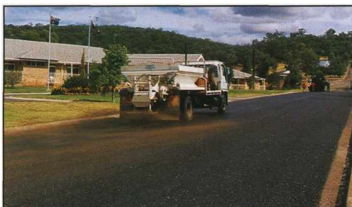
A fine cover of sand is placed by a specialised spreading vehicle to enable early traffickability.
