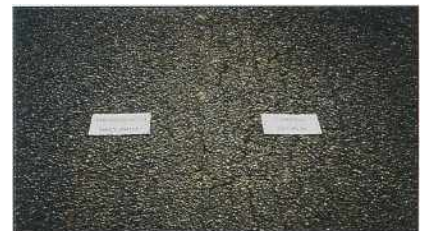
The Reclamite "A" treated surface (left) on Gidgee Street has lasted well, while the control section is showing severe ravelling and cracking.
