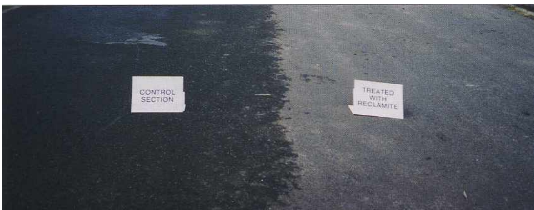
The difference in the permeability of the non-treated (left) and treated sections of pavement on Rickard Road can be clearly seen in this photo taken after light rain.
