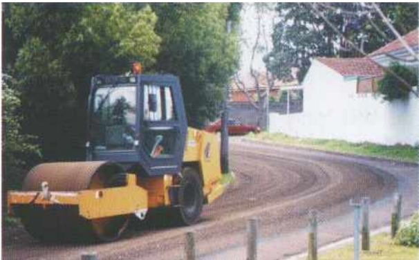
The PolySeal Process produces superior stone retention which allows sweeping on completion of rolling, minimising loose stone issues.
