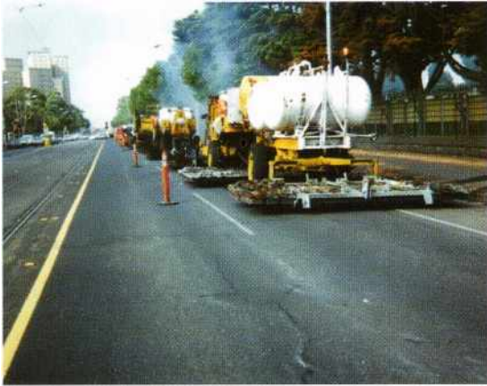
Lygon Street Melbourne, showing cracking and asphalt deformation.
