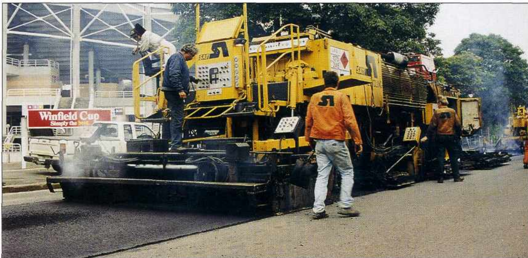
For larger areas, SAT has a HIPAR machine which can recycle and pave up to 4.5 m wide in a single pass. The application above shows Moore Park Road, outside the Sydney Football Stadium, being recycled using the HIPAR process on behalf of South Sydney Council.
