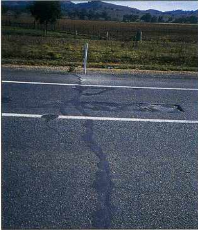
Left: The extent of cracking on the Hume Highway prior to treatment with GlasGrid and AC overlay. Above: The paving process.
