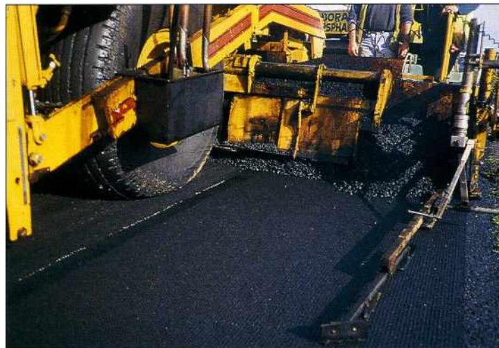
The AC wearing course being placed over GlasGrid.
