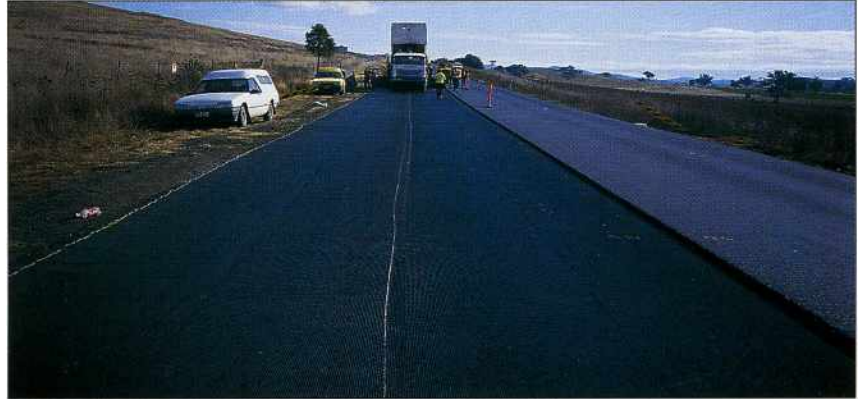
Left: The extent of cracking on the Hume Highway prior to treatment with GlasGrid and AC overlay. Above: The paving process.
